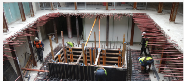
The new stair core coming up through the existing floors
